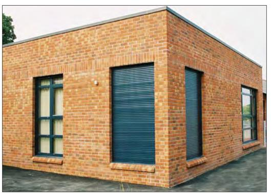
In total 40 shutters were installed at the Sure Start Centre, effectively securing all accessible windows. They were finished in dark blue/ green paint to exactly match the specified colour of the windows.
