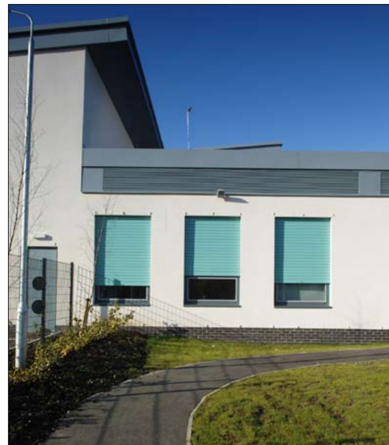
Newark Primary School, Port Glasgow, Scotland (2008): This building enjoys a prominent position in the local landscape and the use of Charter-Integr8 shutters is an important part in the bold and striking design of the school. In this instance perforated shutters were used to allow natural light to enter the classrooms when the shutters are closed.
