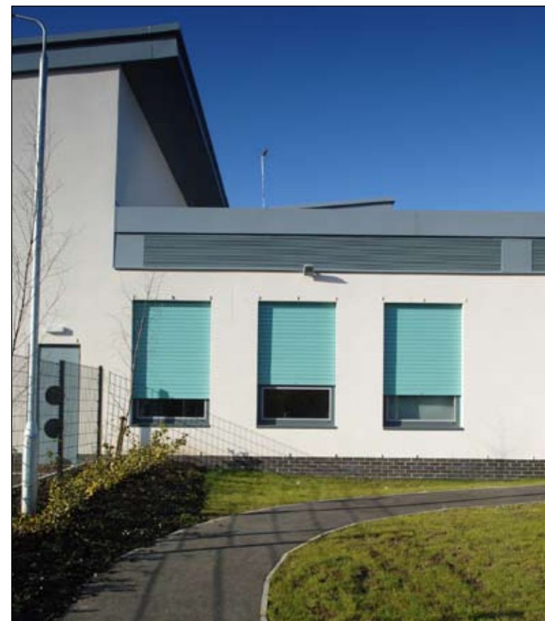
Newark Primary School, Port Glasgow, Scotland (2008): This building enjoys a prominent position in the local landscape and the use of Charter-Integr8 shutters is an important part in the bold and striking design of the school. In this instance perforated shutters were used to allow natural light to enter the classrooms when the shutters are closed.
