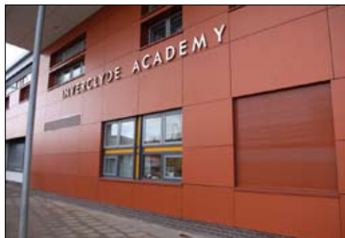
West Inverclyde Academy, Greenock, Scotland (2008): The extensive support offered to clients at every stage of the design and installation process was one of the reasons why Charter was awarded this prestigious contract.
